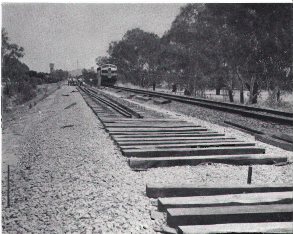
[Victorian Government Railways. Track laying for the new standard gauge line between Melbourne and Albury.
